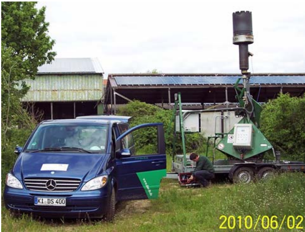
Figure 5 – Mobile flare system on site
